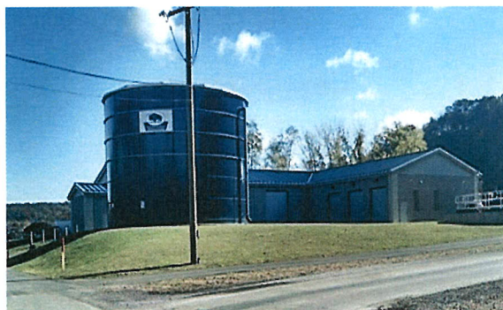
The Stanley K. Swank Freeport Filter Plant
